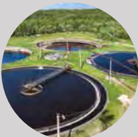
Sewage Treatment Plant for aeration
